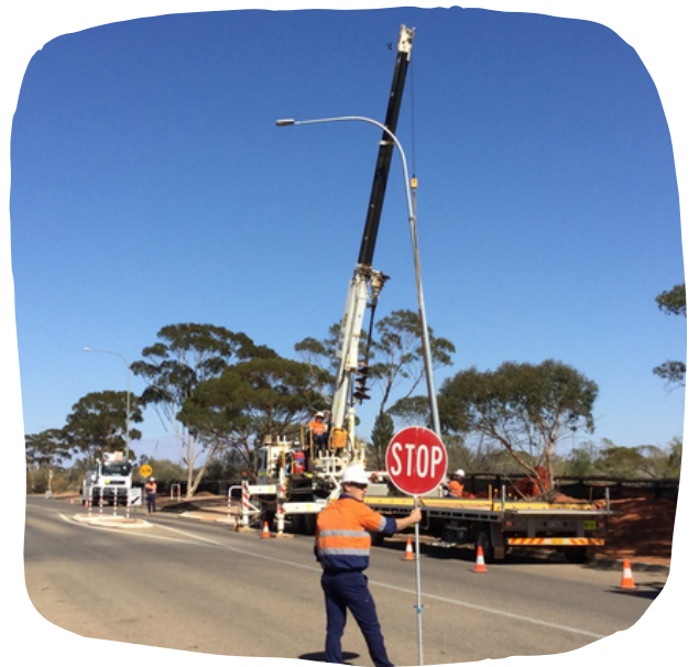
Replacement of a street light on Tutop Street.
