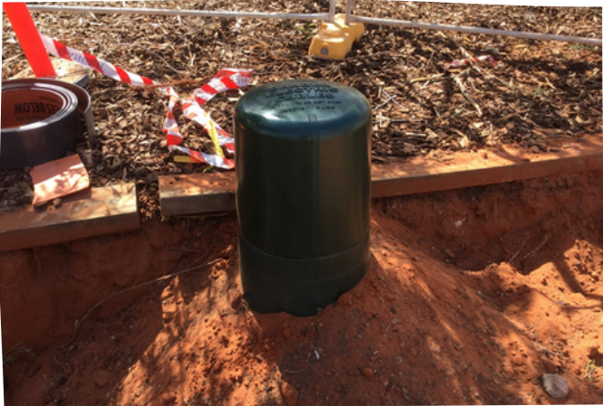
Replacement of service pillars, before and after.
