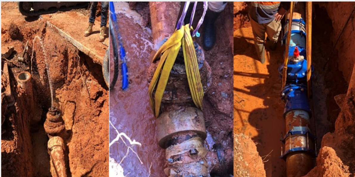
Replacement of the water mains isolation valve.
