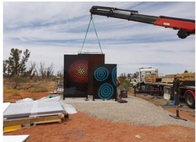
Installation of the Town Entry Statements.
