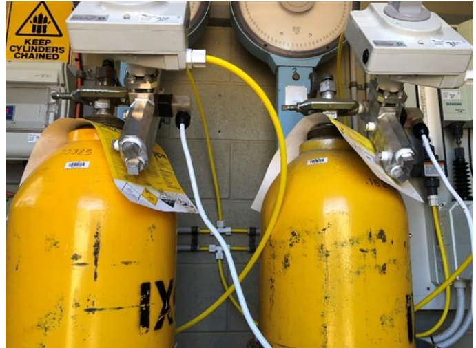
Drip legs on the chlorine dosing system.
