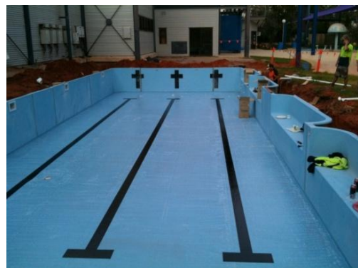
Indoor Aquatic Facility under construction
