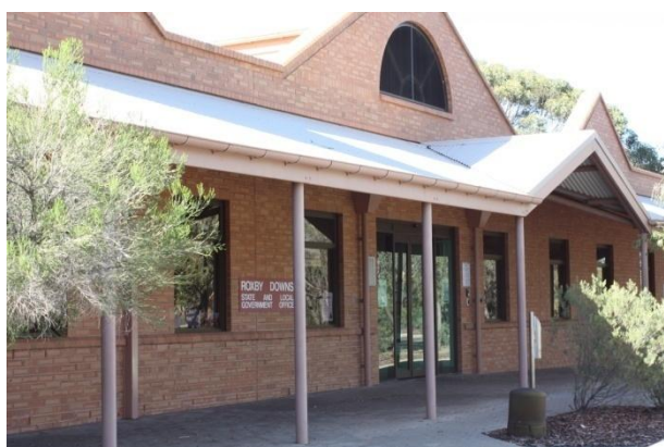
Roxby Downs Council Offices in Richardson Place
