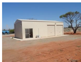
New Storage shed at the Township water supply Built as storage for generator trailer and crane trailer. Also toilet and work area.
