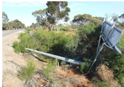
Vehicle damage to a street light on the end of Pioneer Drive.
