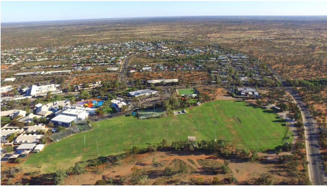
Aerial view of Town Ovals and Roxbylink complex
