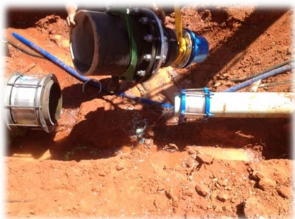
Water Main repair
