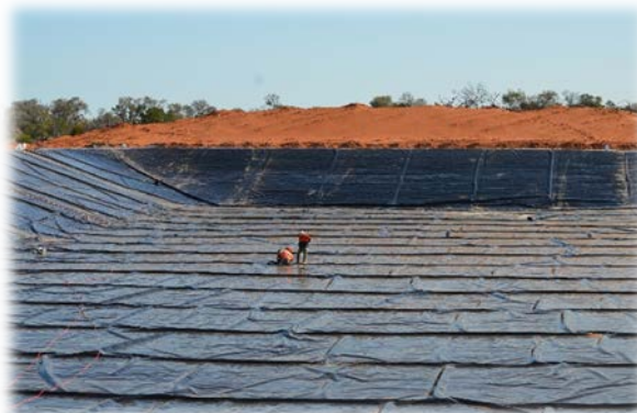
Lining of the new winter storage dam at Sewer Lagoons
