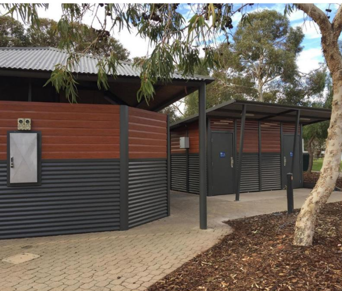
RICHARDSON PLACE TOILETS
