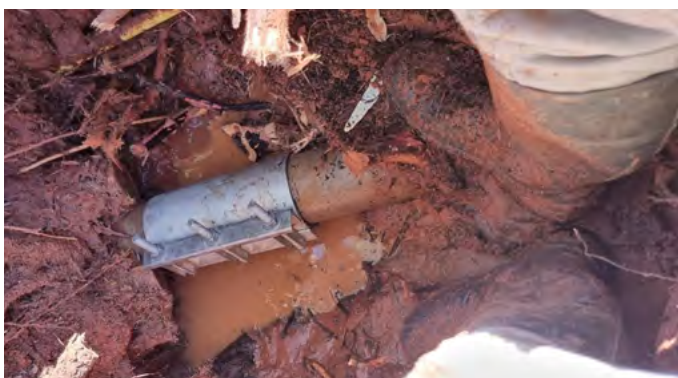
Water Mains Repair on Mirra St Stainless Steel Repair Clamp
