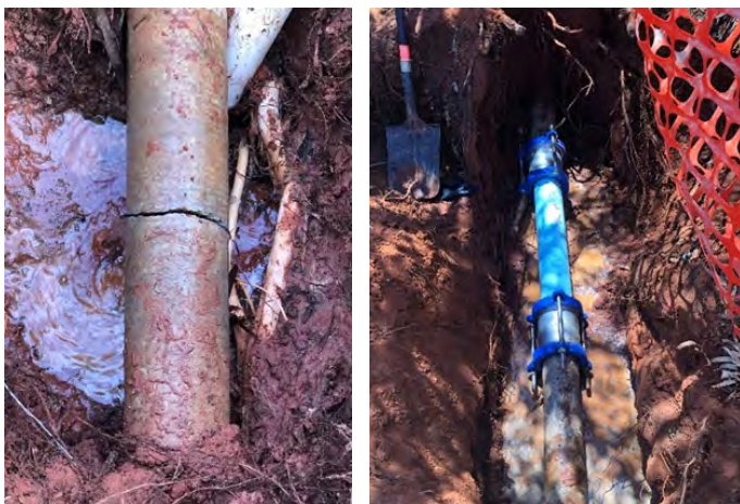
Repairs to Water Mains Leak Wangianna St October 2022
