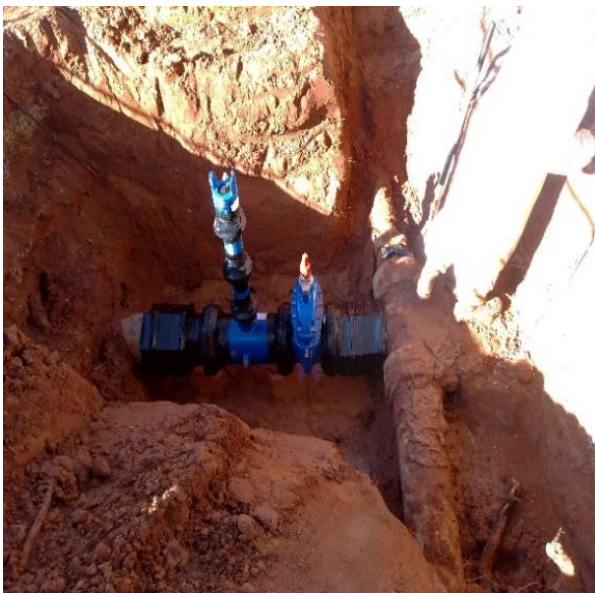
New isolation valve and fire hydrant, Pioneer Drive.
