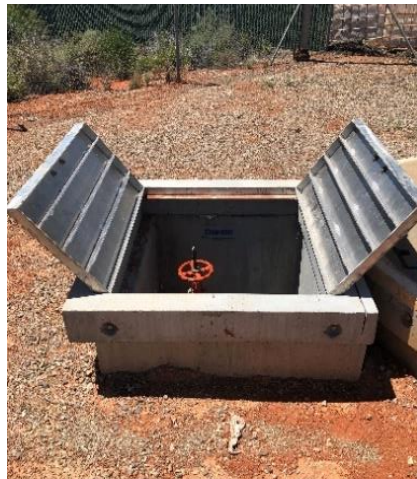
New non-return valves and concrete pit at Pump Station F
