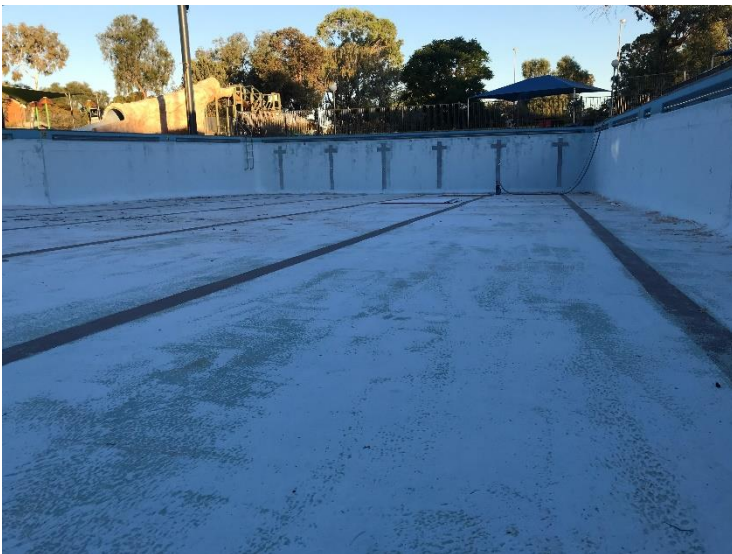
Resurfacing the main pool
