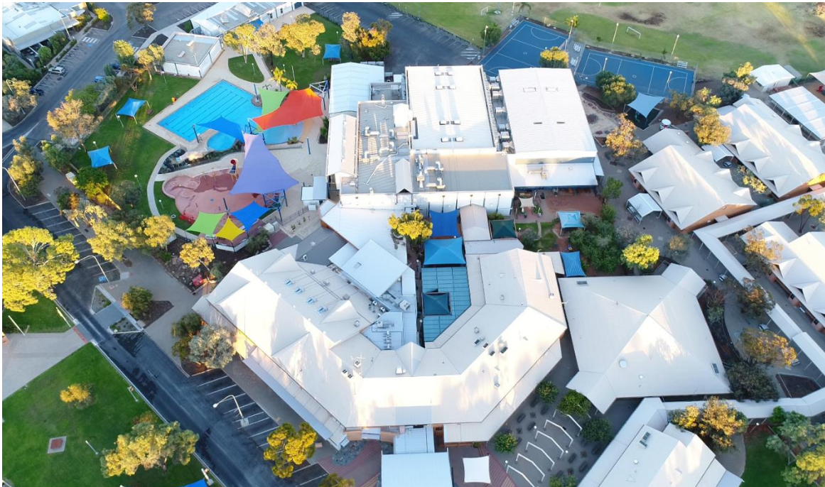
Aerial view of the Roxbylink Cultural and Recreation complex
