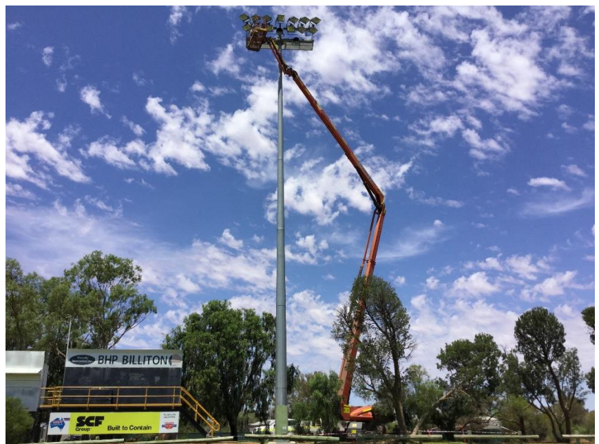
Maintenance of the oval lights
