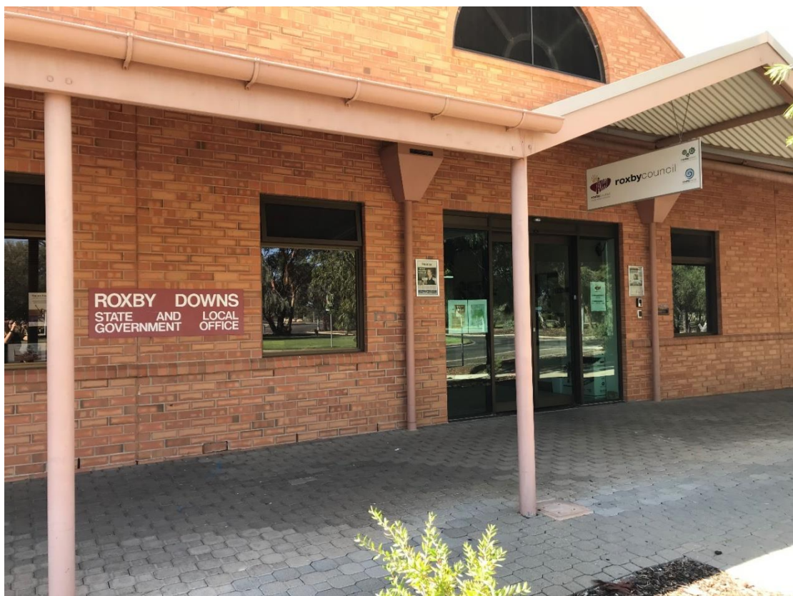
Main Council Office in Richardson Place
