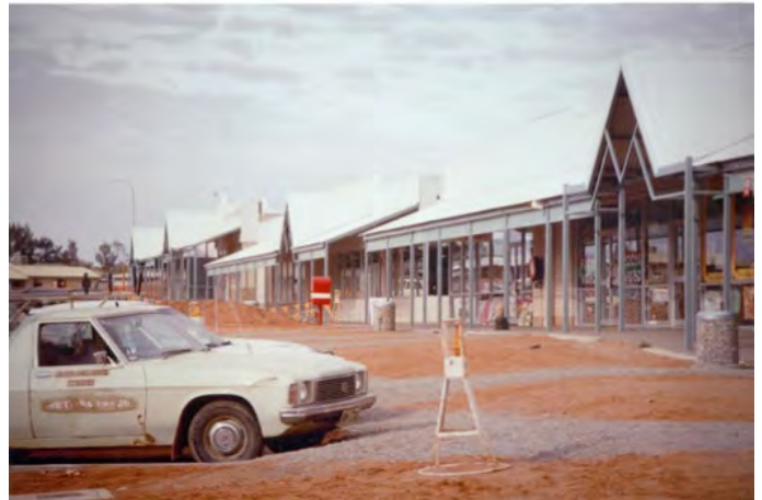
Richardson Place Construction circa 1987/1988 (source Travis Hague)
