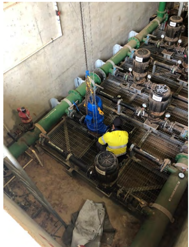
Installation of new pump at the Town Water Supply
