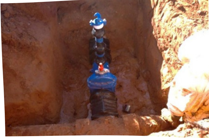
New isolation valve and fire hydrant on Pioneer Drive.
