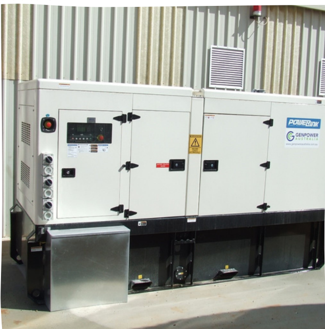
Installation of the new 200 kVA backup genset.
