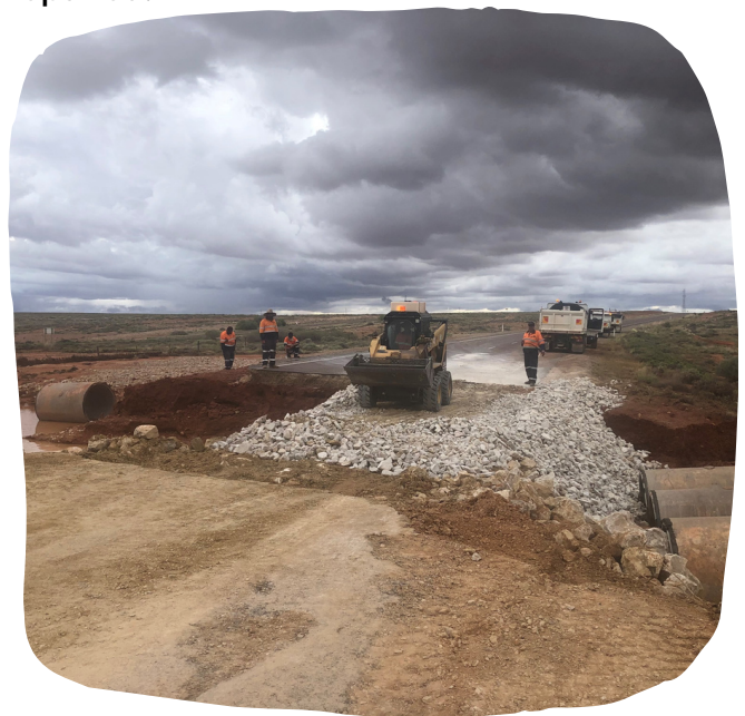
Contractors at work rebuilding the road that was washed away.
