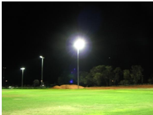
New Lighting erected at the Small Oval
