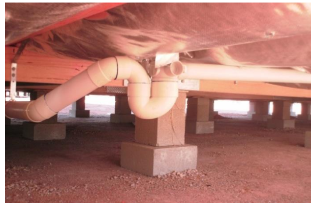
Underfloor inspection of new house
