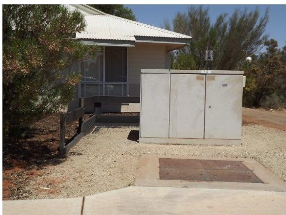
One of several landscaping projects, in this case to provide adequate working clearances and drainage.
