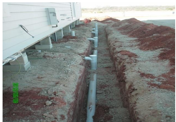
Connections to main drain inspections
