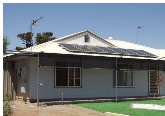
One of many new SOLAR Systems installed in Roxby Downs since September 2011.
