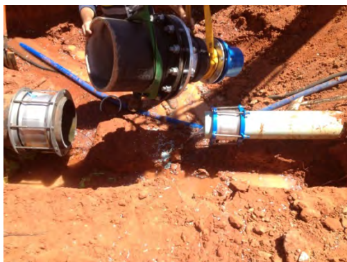
Water Main repair – Olympic Way
