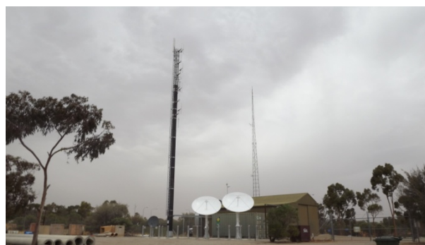
New digital TV tower and satellite dishes, also has Radio antenna. Transmission equipment facility is within the Depot shed
