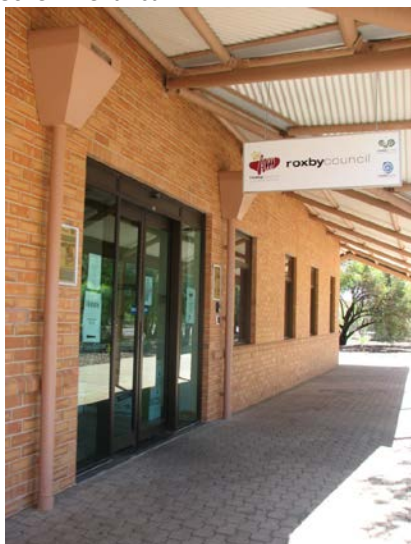
Roxby Downs Council Offices in Richardson Place
