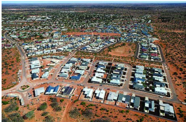
Aerial view of new developments
