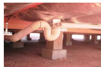
Underfloor inspection of a new house
