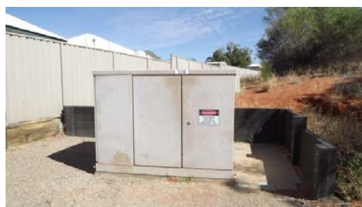
One of several landscaping projects, in this case to replace a failed retainer wall.
