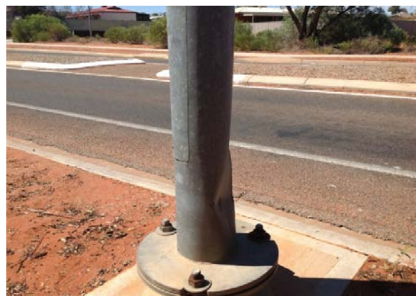
Street light pole damaged by vehicle was replaced.
