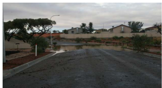
Some damage occurred and was soon repaired
