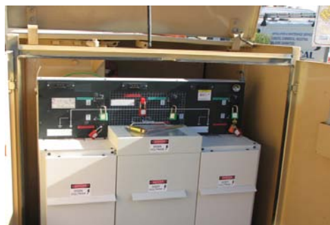
Replacement RMU installed at Roxby Downs Caravan Park
