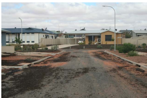
This happened on the 8th April 2010 when approximately 130 mm fell in a very short time and flooding areas in the township that drained away very quickly
