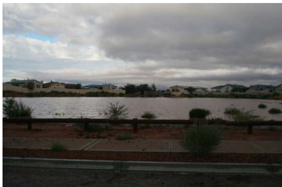
The storm water system has been built so that some roads become the water carrier in large intense rainfall events
