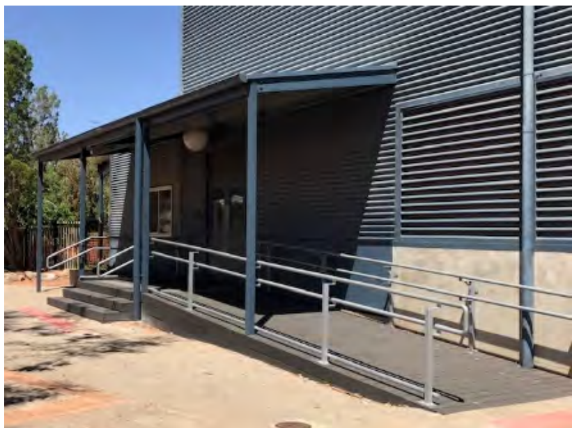
New ramp at Stadium Two
