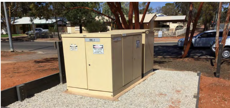
Transformer upgrade on Pioneer Drive
