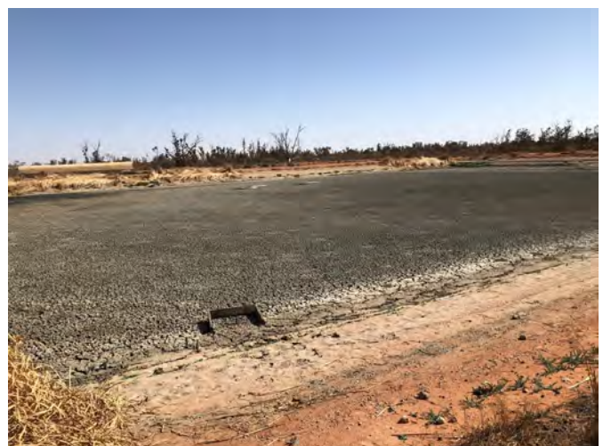
Sewer lagoons during desludging process
