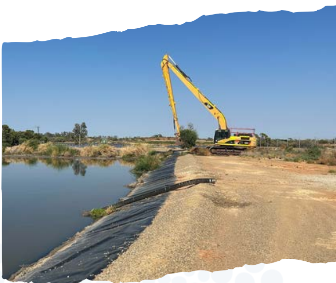
Reeds and Weeds at the anaerobic Dam (Sewer Lagoons)
