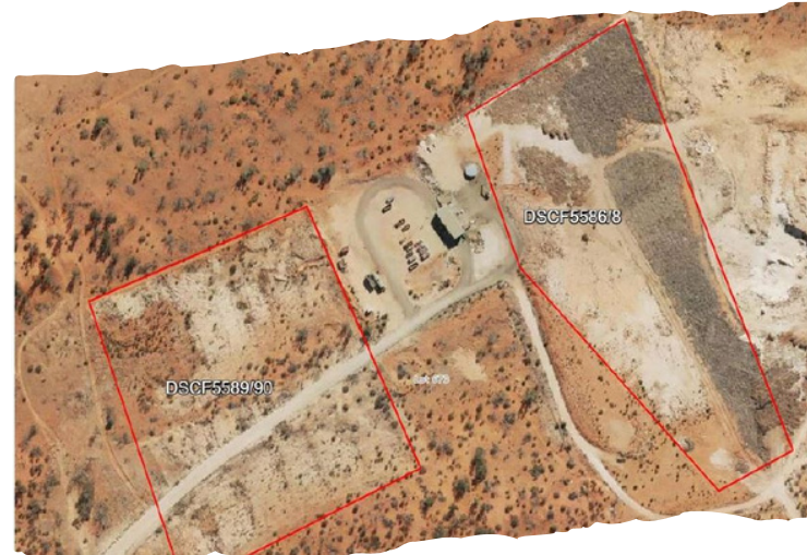
Image 3 - Opal Road Waste Management Facility Landfill cells (footage taken circa 2018)
