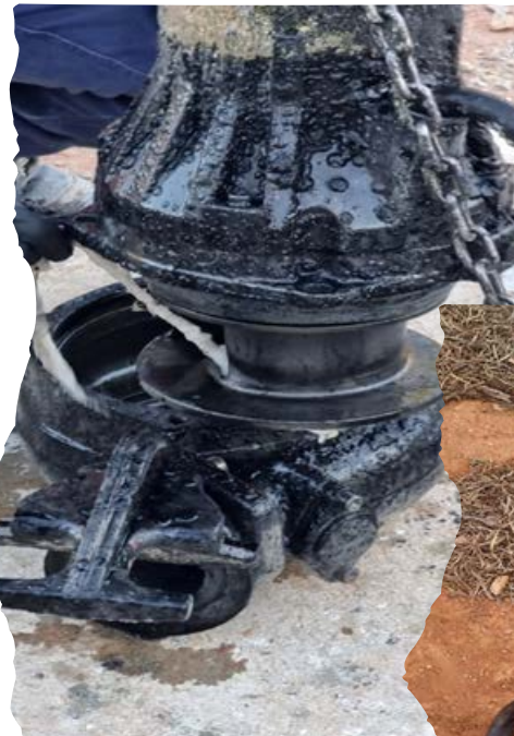
Lift and Clear a Pump at Pump Station E
