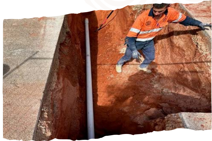
Replacing a section of Sewer Mains on Blanche Court
